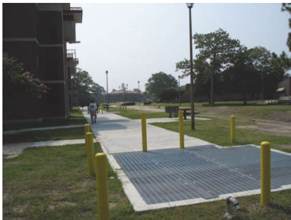
Figure 4.6 Manhole with an open grate cover.
