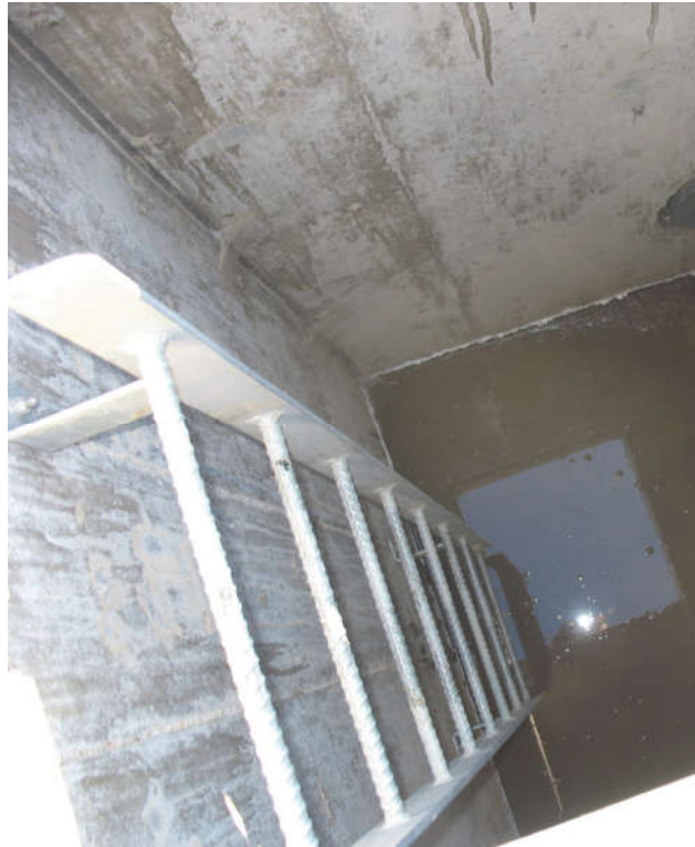
Figure 4.8 Steel manhole ladder, hot dip galvanized after fabrication.
