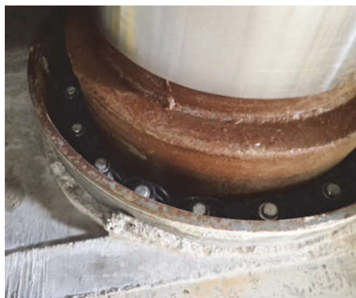
Figure 4.5 Rubber seal between outer pipe casing and steel sleeve through conduit wall. Bolts are tightened to compress seal in annulus.
