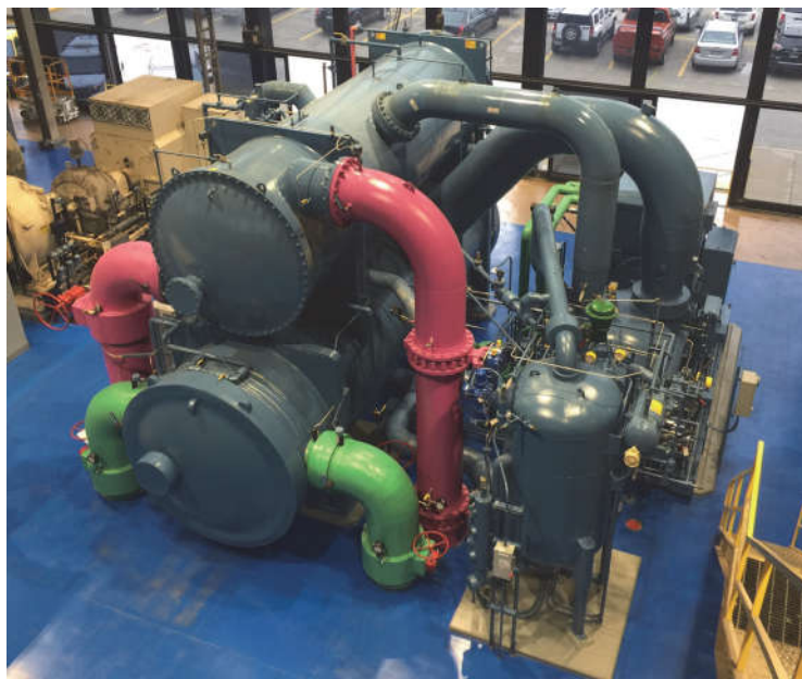
Figure 3.2 4500-ton, field-erected electric- (4160V/60 Hz) driven chiller (HFC-134a). Photo Courtesy of Burns & McDonnell Engineering Company, Inc
