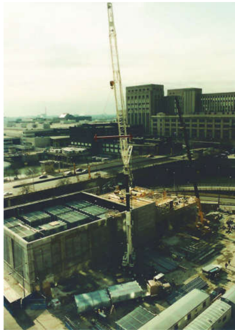
Figure 6.1 The 125,000 ton-h (440,000 kWh) of ice-on-coil TES at Enwave Chicago's District Cooling Plant #2 in Chicago, Illinois, was first in-service in 1996. The 114 ft long × 91 ft wide × 32 ft high (34.7 m × 27.7 m × 9.8 m), 2.5 million gallon (9400 m 3 ) concrete tank, holding 144 ice-on-coil modules, operates at a nominal water-glycol charging (ice building) temperature of 20.5°F (−6.4°C), and a water discharging (ice melting) temperature of 34°F (1.1°C). It can reduce peak demand by up to 14,600 tons (51,000 kW) of cooling and approximately 10 MW of electric power.
