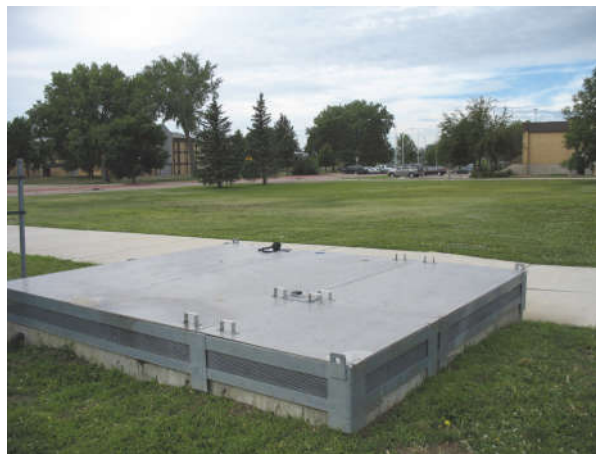
Figure 4.7 Manhole with a raised cover and vented sides.
