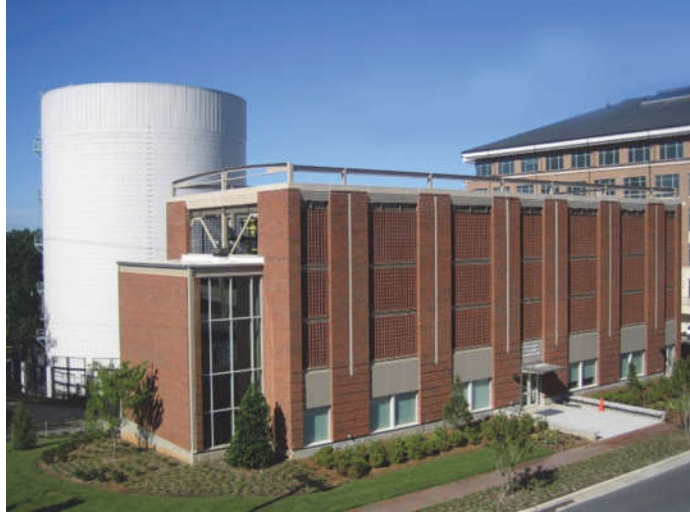
Figure 6.8 The 40,000 ton-h (140,000 kWh) of stratified CHW TES at the University of North Carolina in Chapel Hill, North Carolina, was first in service in 2004. The 85 ft diameter \times 116.83 ft high (35.6 m \times 25.9 m), 5.0 million gallon (18,800 m 3 ) welded-steel tank, operates at CHW supply temperature of 41°F (5°C) and a return temperature of 54°F (12°C) and was designed for possible future conversion to LTF TES service at a larger \Delta T and increased thermal capacity. In CHW TES service, it reduces peak demand by up to 10,000 tons (35,000 kW) of cooling and approximately 7 MW of electric power (or approximately 40% higher if converted to LTF TES).
